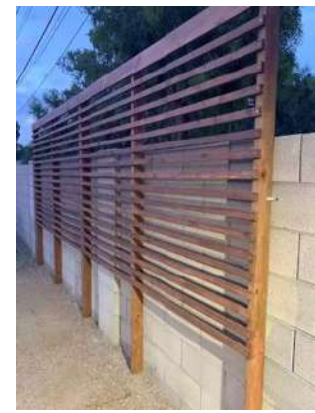
Figure 80. Concrete fencing wooden plank panels
